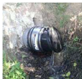
MULTI N valves installed on banks, PVC pipes
