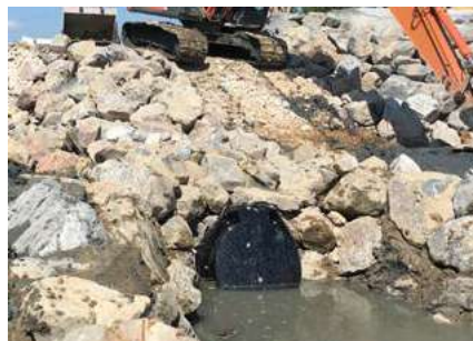
MULTI NB valves installed on banks
